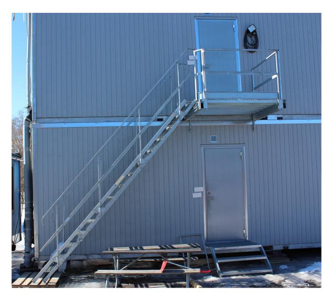
Completely mounted access route for upper floor, here with HP2001 - 15 Steps staircase, which is our shorter / steeper variant, so that the stairs will not protrude outside the lower barack.
