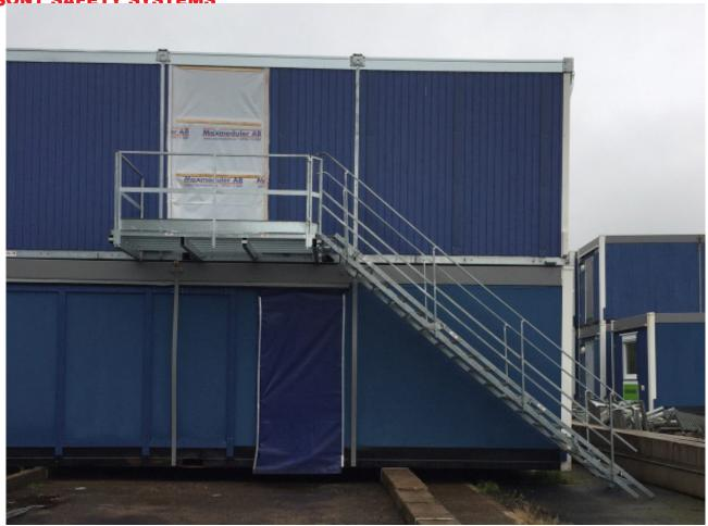
Completely mounted access floor for upstairs housing, here with HP2000 - 18 Step living staircase which is our longer variant.
